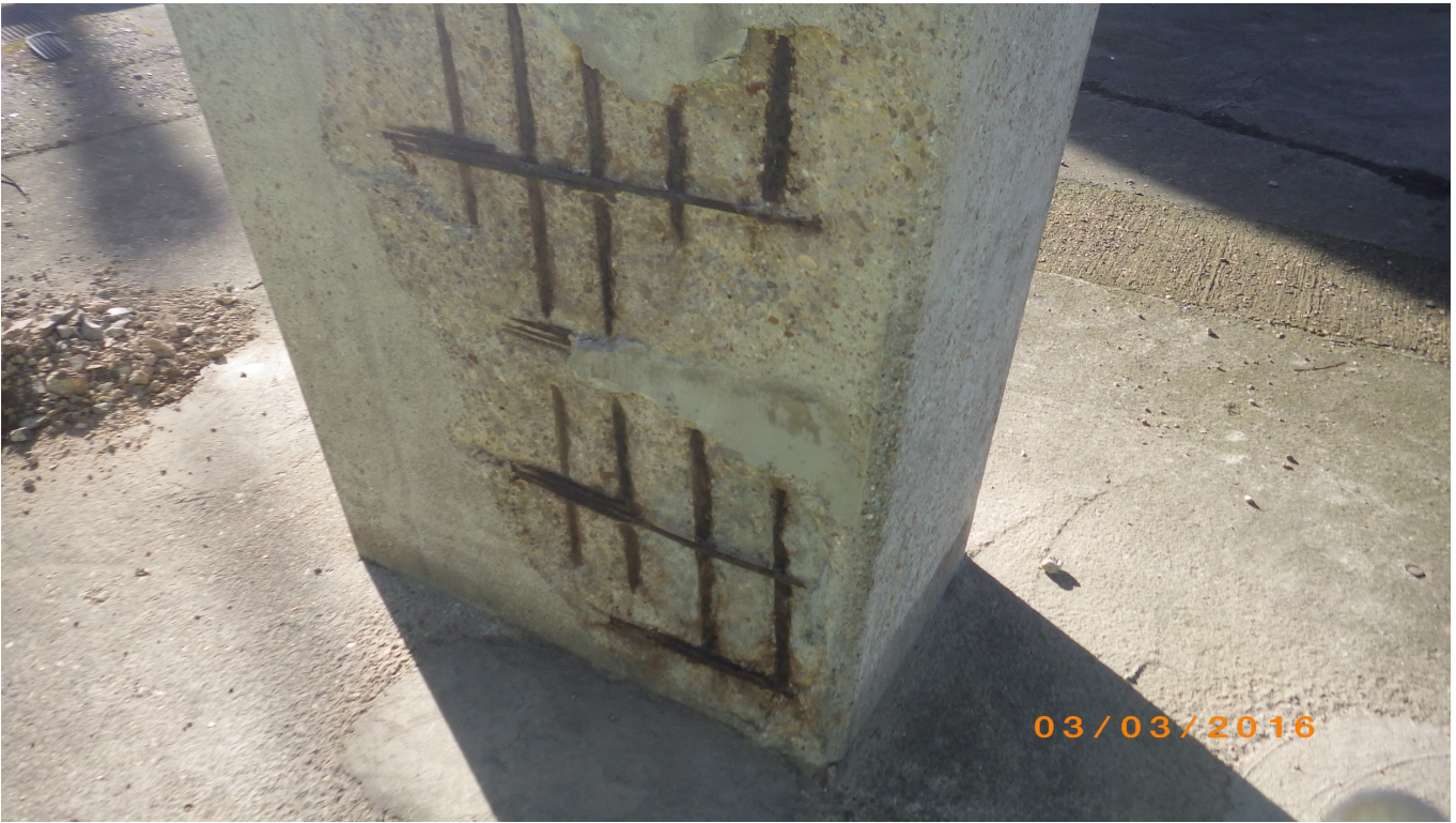
Figure four: Sheets of poor concrete have spalled from the piers exposing the corroded reinforcement
