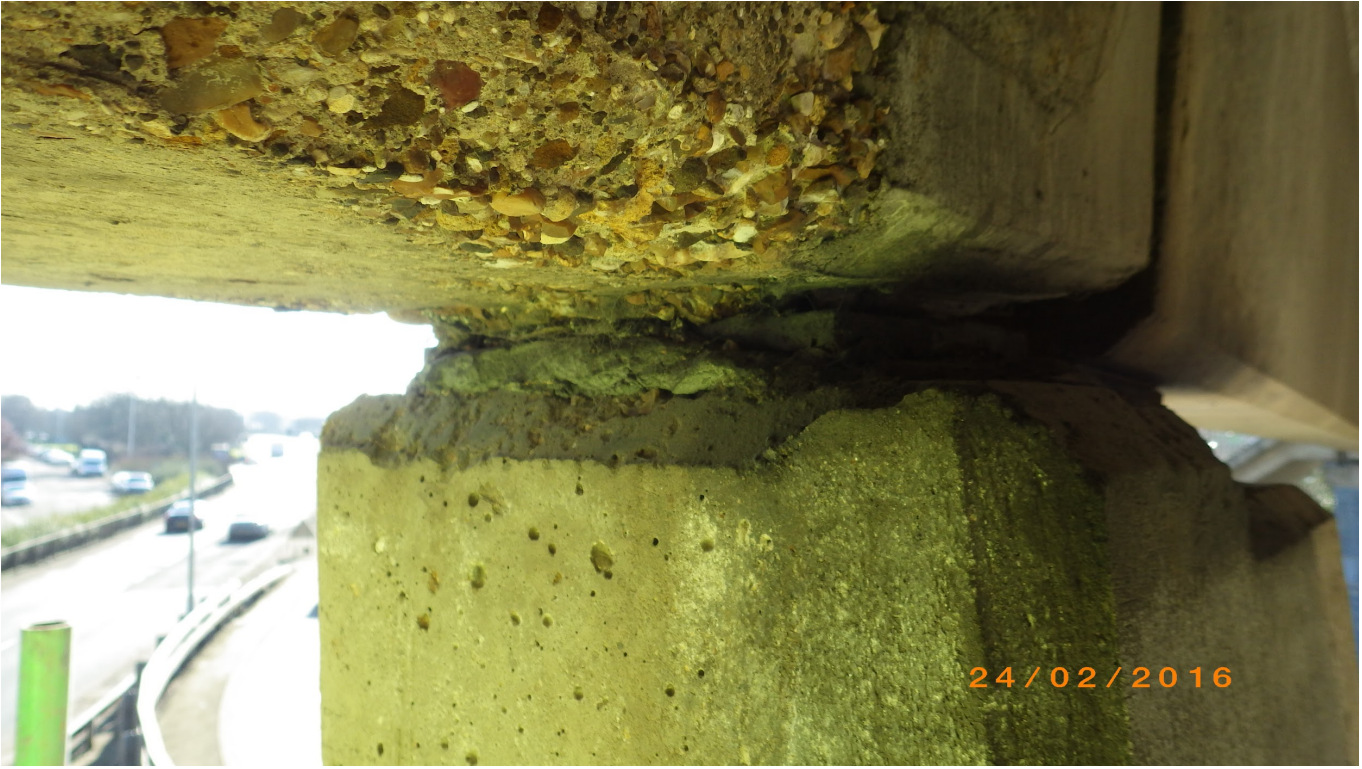
Figure four: Sheets of poor concrete have spalled from the piers exposing the corroded reinforcement
